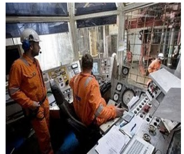
Control room operations monitor hazardous liquid and natural gas pipelines through computer equipment that records and displays operational information.
